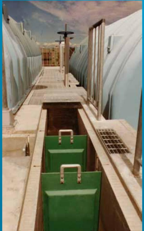
The Plasti-Fab Light Weight Composite Stop Gate is the ideal solution for corrosive environments that cause metal gates to seize or freeze in place. Composite Gates have no chemical bonds that may brake down and cause the gate to fail. Plasti-Fab Composite Stop Gate installations are still in operation after over 40 years and continue to operate and function as designed.
