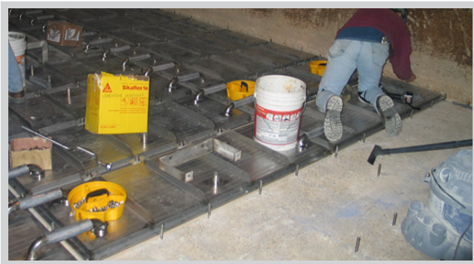
Phoenix™ Panel installation in progress. Time required is 3 days.
