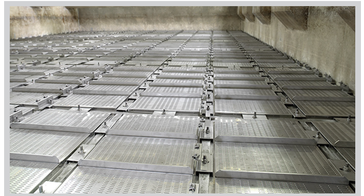
Phoenix™ Panel installation complete.
