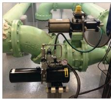
**In-Conduit Energy Recovery**The Granville Pipeline and Hydroturbine installation for the City of Westfield will take advantage of in-conduit energy recovery to supply up to 37 kW.
