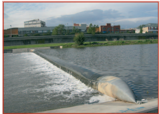
⬆️ Rubber dam on River Besos near Barcelona.
