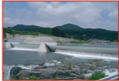
✓ Two 45m long rubber dams at Kagoshima in Japan.
