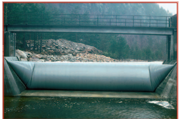
Ⓥ Sumitomo Electric rubber dam in Japan.
