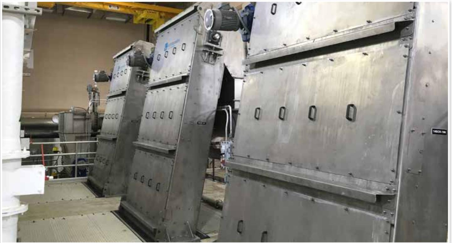
The Kusters Water ProTechtor® Multi-Rake Bar Screen combines fine or coarse screening with high solids capture rates. Its robust construction and overload feature ensure reliable operation.
